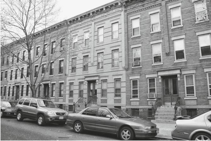
FIGURE 4.3 There are numerous apartment buildings in Bushwick like the ones that appear in this photograph without off-street parking. Indeed, the majority of automobile owners park in the street and constantly move their cars because of street cleaning. Parking late in the evening and at night becomes a difficult undertaking because there is not enough street parking. Reflecting the demographics of the area, the great majority of these car owners are Latinos and African Americans.
