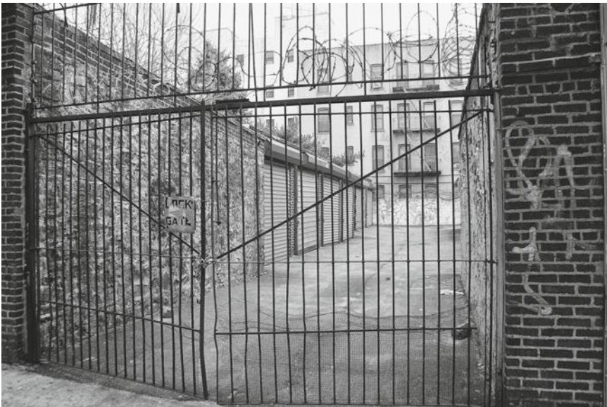
FIGURE 4.2 A series of off-street garages in Bushwick, Brooklyn. With real estate values being low for many years, space was reorganized to accommodate the automobile.
